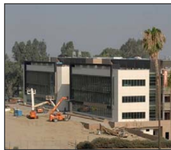
...to a state-of-the-art teaching and learning environment (Centennial Complex)
